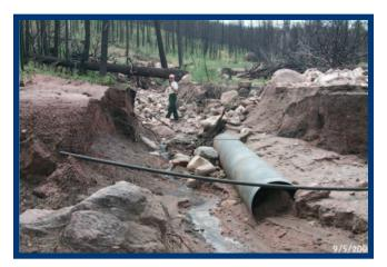
**Figure 10.11**—Rocky Mountain Research Station Engineer Joe Wagenbrenner surveys a channel scour, following the Hayman Fire, 2002, Pike-San Isabel National Forest near Deckers, CO. (Photo by A. Covert).
