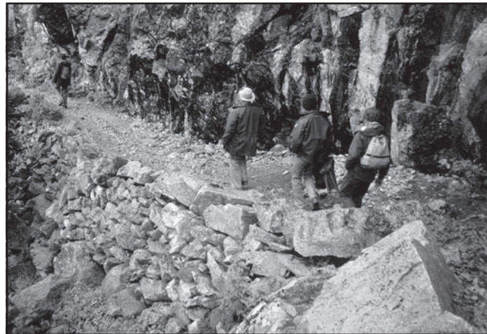
Figure 73—A rock retaining wall is needed to hold compacted fill.
