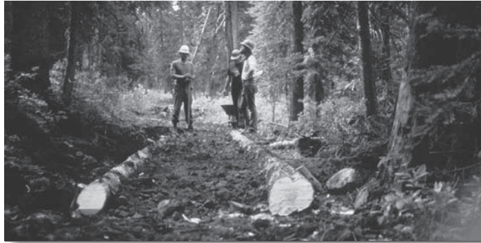
Figure 54—Subsurface puncheon covered with soil and rock.
