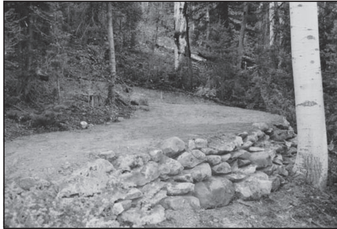
Figure 69—Part of the lower approach and the lower half of this switchback are constructed on fill.
