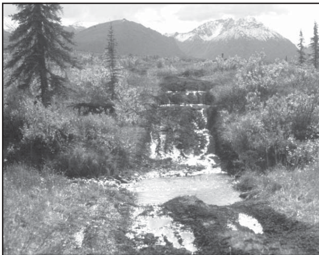
Figure 1—A degraded trail in interior Alaska. Heavy use has stripped surface vegetation and exposed permafrost soils to accelerated melting, resulting in muddy, rutted trail surfaces, erosion, and deep muck holes.
