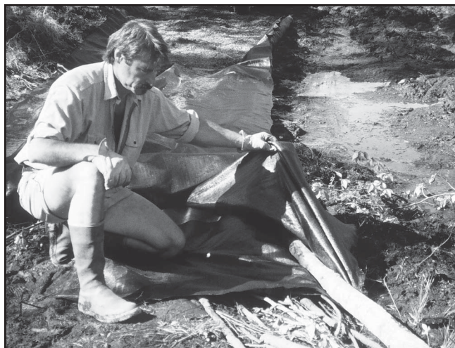
Figure 11—The author installing woven geotextile around a rim log in the geotextile gravel-capping test installation at the Yukon-Charley Rivers National Preserve in Alaska. The rim log held the gravel cap on the installation.
