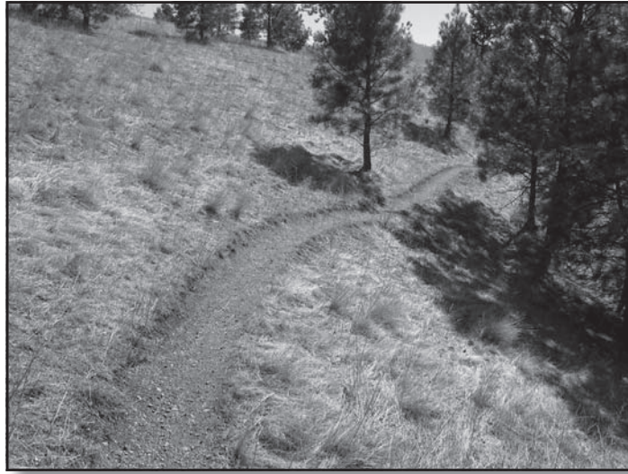
Figure 1—A rolling contour trail resists erosion.
