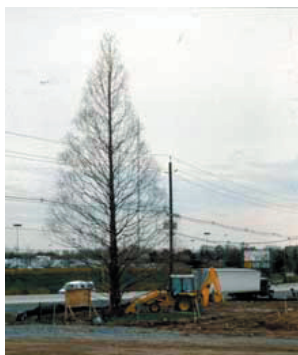
Figures 3.83-3.84. To estimate how much root damage was sustained, determine how much of the Critical Root Radius was disturbed.
