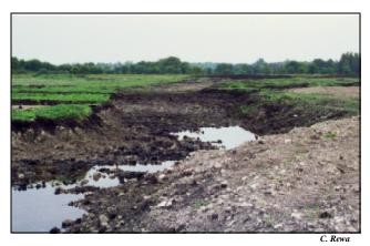
Surface contours can be excavated during the wetland restoration process to increase the diversity of water depths and associated wetland vegetation.
