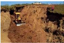
Crawler tractor forming a firm bed for a pipe drop structure.
