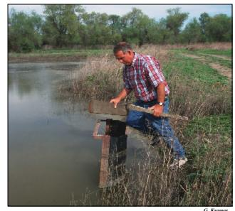
Drop-log inlets and other water control structures can be installed to enable managers to manipulate water levels on restored and created wetlands.
