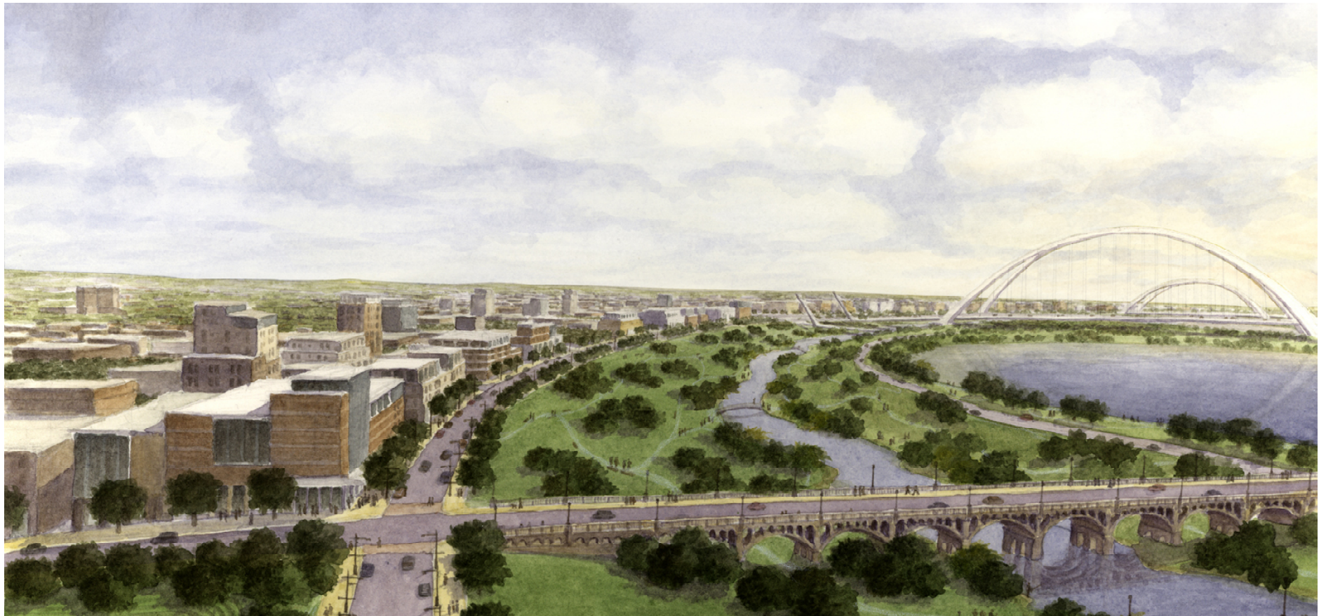
View of the proposed Oak Cliff levee-top road with future development along it. In the foreground is the Houston Viaduct. The Calatrava Bridges are in the background.
