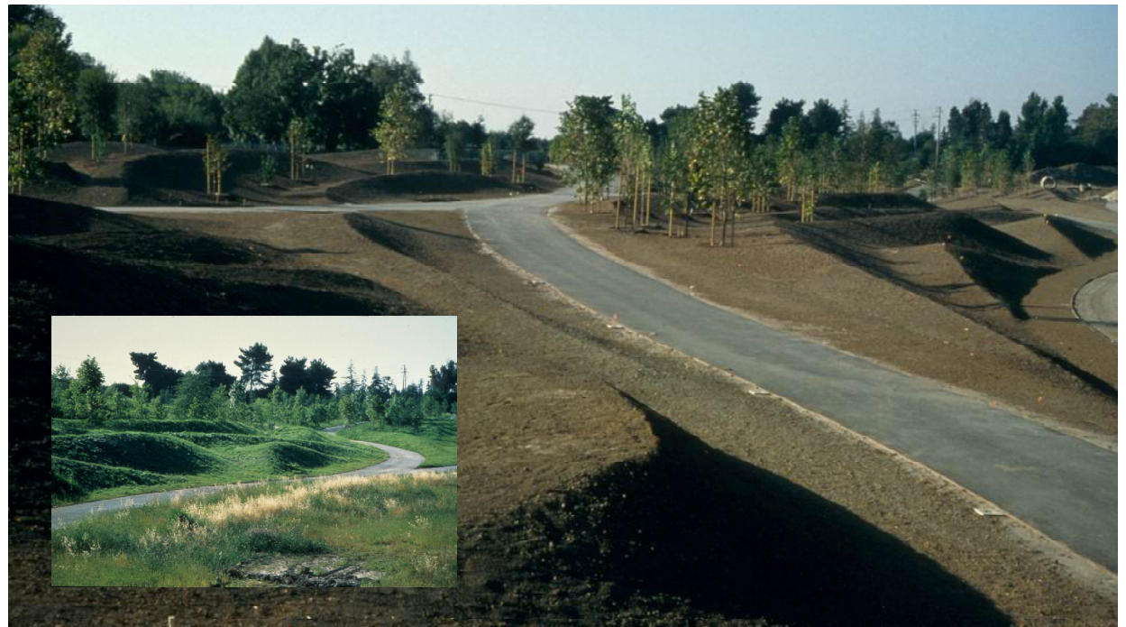
Landforms can be used to manage or “fine tune” floodway performance by slowing or redirecting flows.
