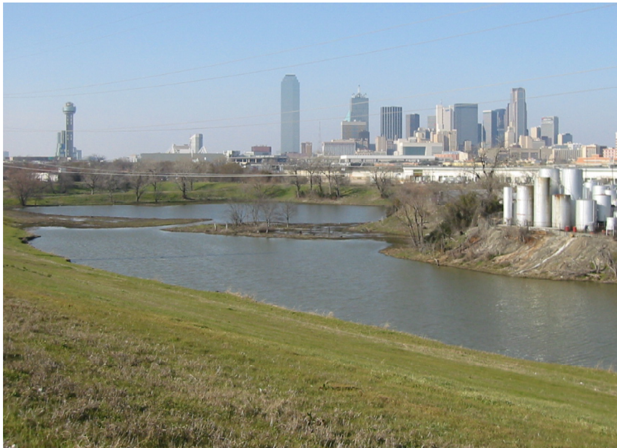
Preserving existing valley flood storage: the “sump” at Cedars West.
