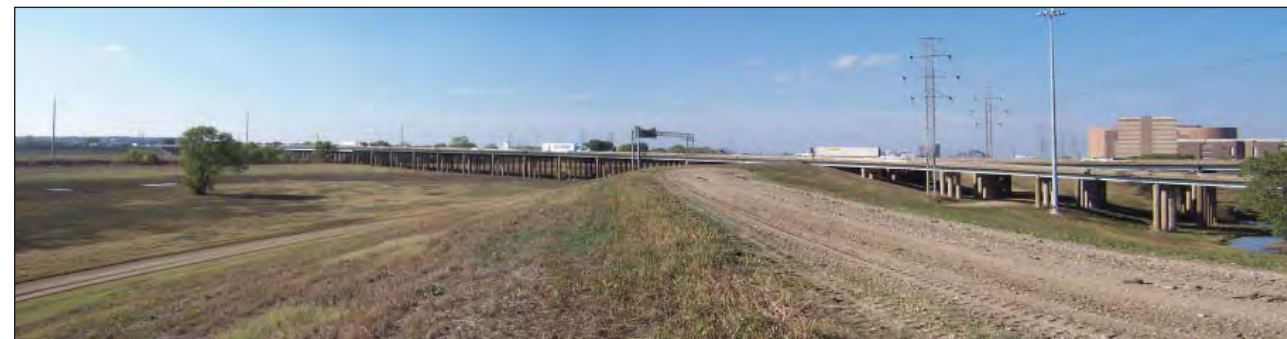
4: View from 1238+00 looking North toward IH-30
