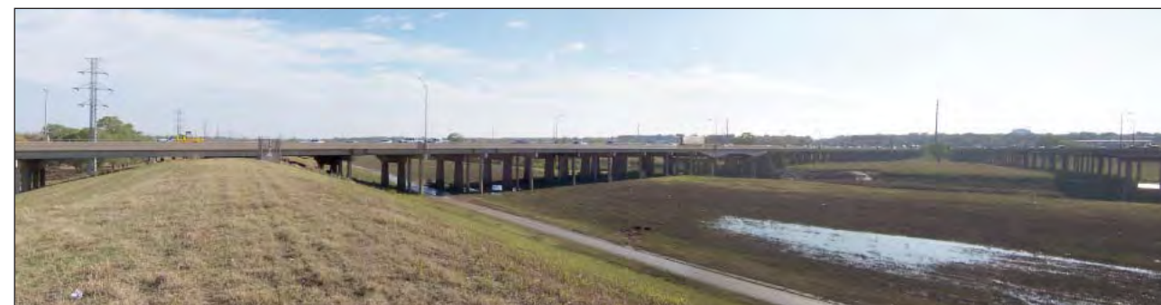
6: View from 1267+00 looking South toward Northbound IH-35
