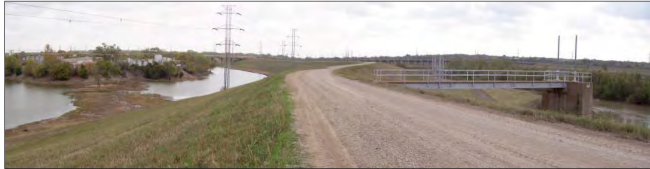
1: View from 1289+00 looking South
