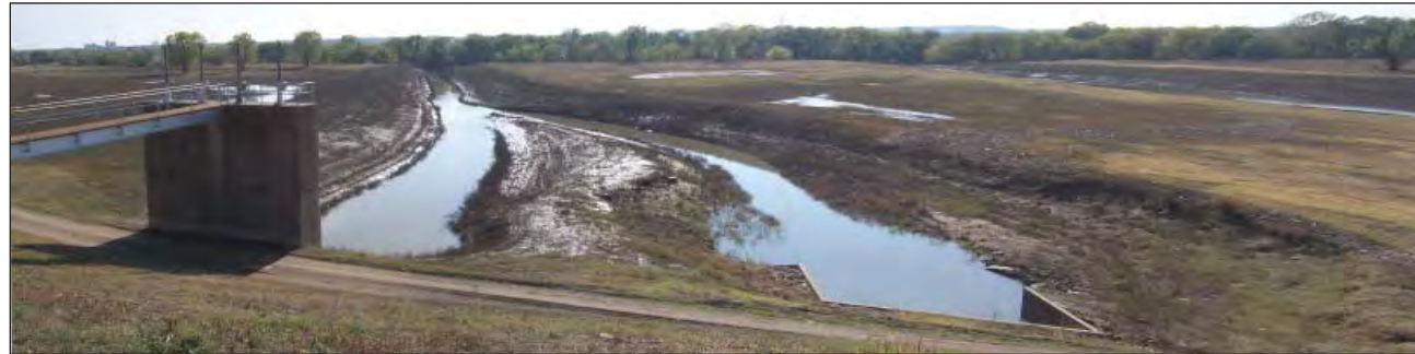
2: View of 1114+00 Pump Station looking West
