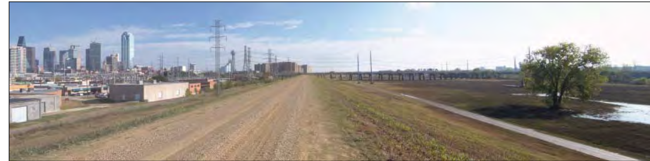
5: View from 1171+00 looking South toward Continental Viaduct
