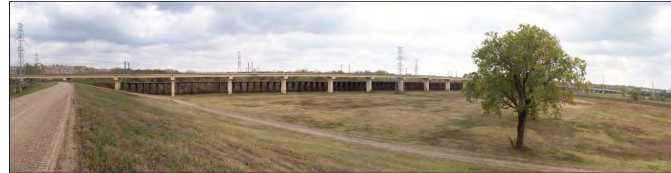
5: View from 1325+00 looking South toward the DART Railway
