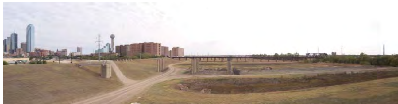
1: View from 1185+00 looking South
