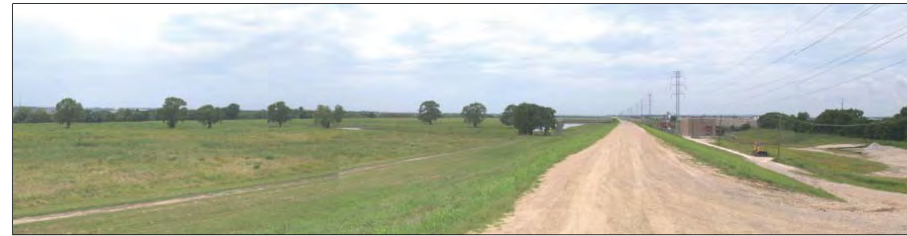
5: View from 1050+00 looking North - Pump Station at right of photo, Westmoreland Bridge in distance
