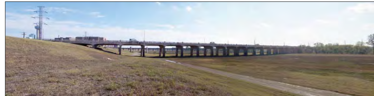
6: View from 1181+00 looking South toward Continental Viaduct
