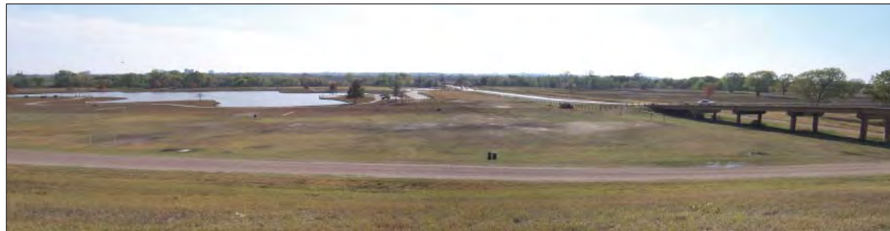
3: View of Sylvan Bridge at 1129+00 looking West
