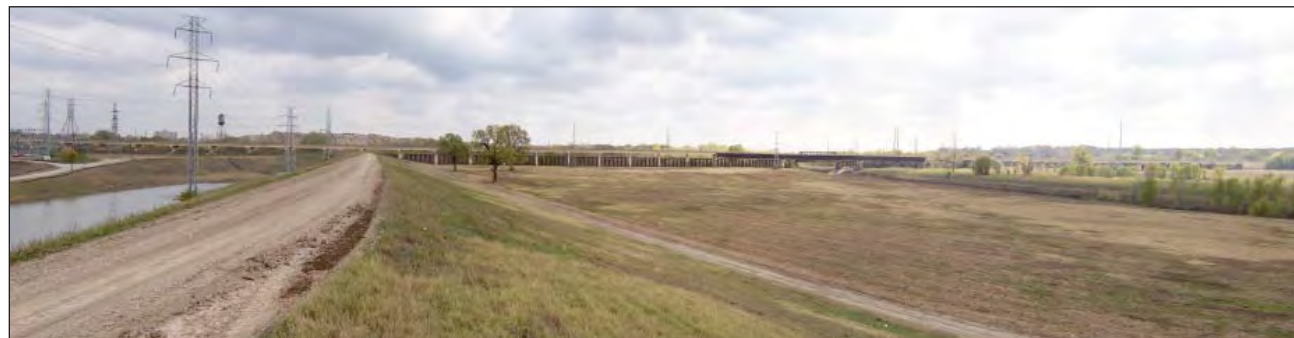
3: View from 1316+00 looking South
